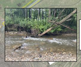
In selected areas with bank erosion, grade streambanks to stable slopes (3:1 or flatter) and reinforce with toe wood revetments as needed; install in-stream structures (log vanes) in these areas for bank protection, flow direction, and improved habitat.
