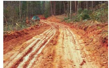
Poorly planned and maintained dirt roads, unstabilized ditches, and road banks are major sources of sediment in Haywood County. Check your erosion controls regularly. If additional measures are needed, install them before you have a major washout.
