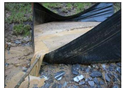
To reduce sedimentation, erosion and sediment control measures must be installed and maintained correctly.
