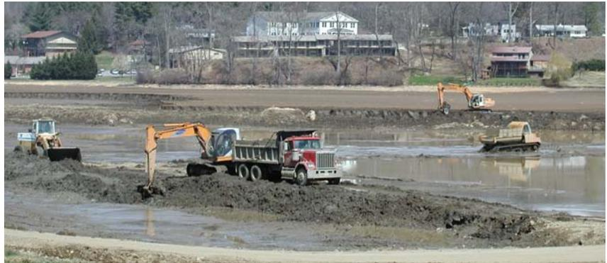
The Lake Junaluska Assembly spends nearly \$70,000 every other year to remove sediment from their lake. This does not eliminate the problem, it only slows the filling rate of the lake. Each year the Assembly removes over 20 tons of debris from booms at the lake entrance (2008 data).
